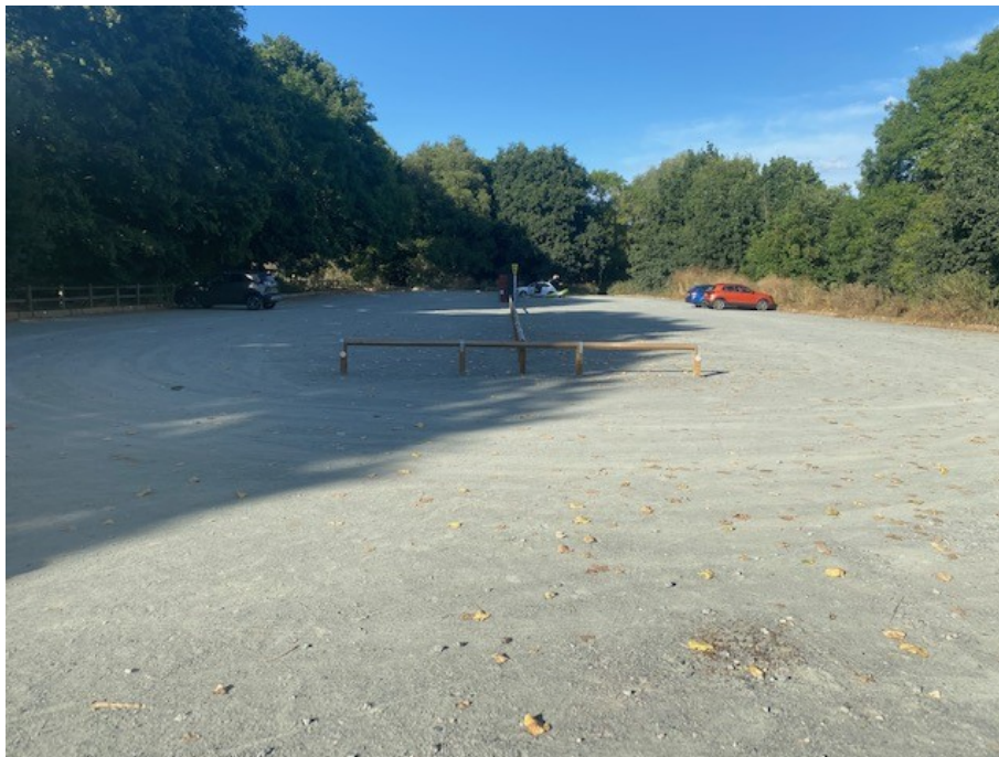
Teston Bridge overflow car park following resurfacing
